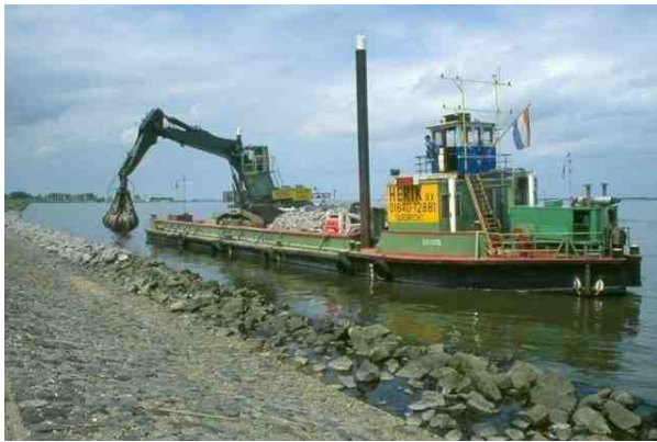
Maintaining wave breakers
